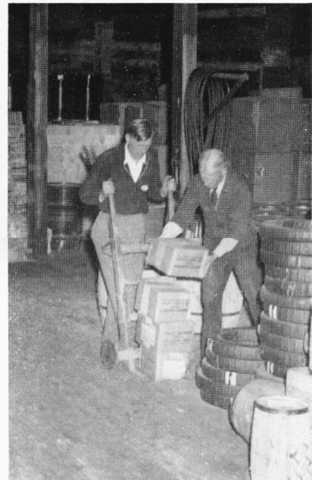
To Store #3, Building 29, come truckloads and carloads of material which are broken up into small lots and prepared for delivery to Scovill Departments. Charlie Pechalonis and John McCabe are old timers at the game of pitching into a carload and making it vanish into an obscure corner in short order. Products of every clime and state are gathered here.
